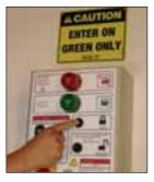
When the trailer is in the parked position, the dock attendant inside pushes the "lock" button on the control box for activating the locking arm assembly. The inside and outside LED lights will change automatically.
